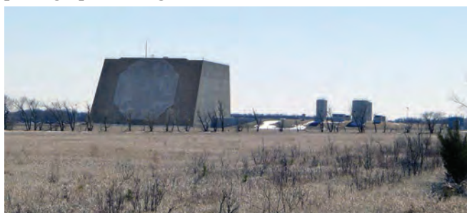
The PAR bunker taken from nearest public road. PAR surface bunker to the left with the underground powerplant and its stacks on the right
